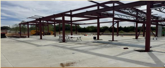
Structural steel and roof trusses erected across the completed concrete pad.
