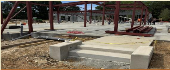
Gable end framed with entry stairs formed — building taking its final shape.
