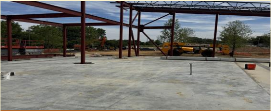
Exterior wall framing going up; crews sheeting the building envelope.
