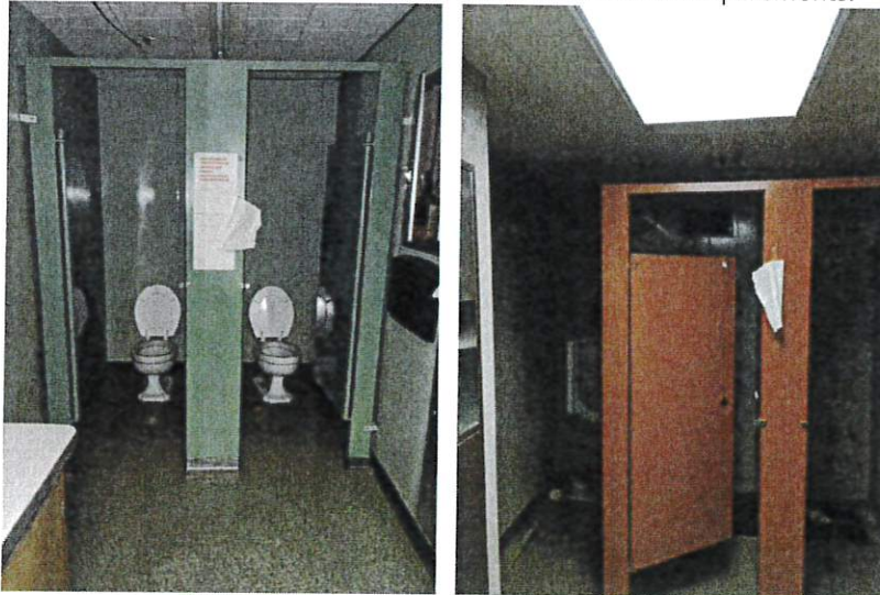
Basement Level Men's and Women's Toilets
