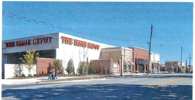
National retail stores can implement adaptive designs and contribute to the character of the community.
