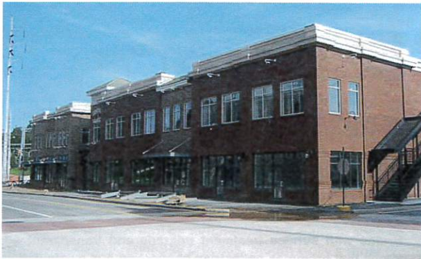
Mixed-use project with building along the back edge of sidewalk and appropriate sill height.
