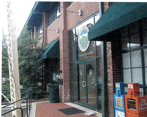
Adaptive re-use of historic structure
