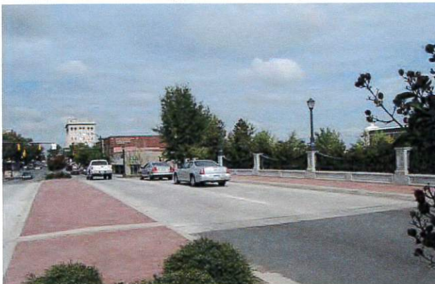
Pedestrian friendly bridge overpass
