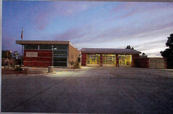
Mount Holly Fire & Rescue Station 35
