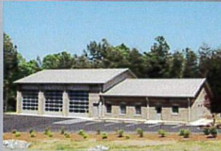
Sherrill's Ford Fire Station 3 Built 2010-2011 $600,000
