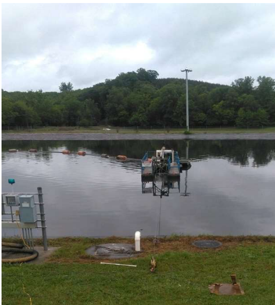
Hydraulic Dredging EQ Basin
