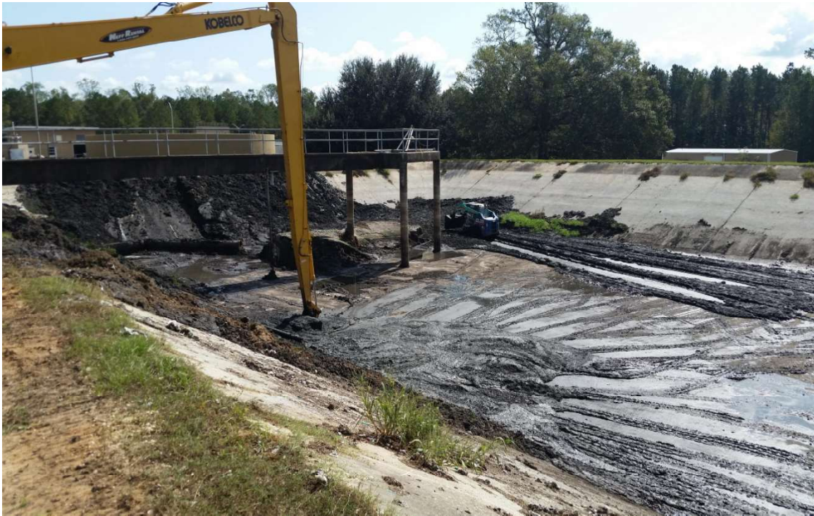
Basin sludge removal – skid steer system, pumping, excavation
