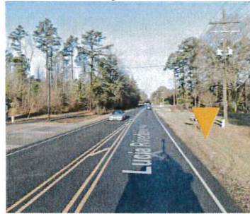
MTI-C HWY 16 East at Lucia Riverbend HWY New Boulevard Scale Sign
