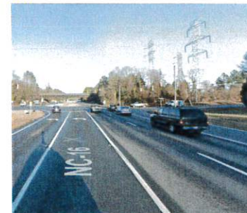
MTI-A HWY 16 West at Lucia Riverbend HWY New Boulevard Scale Sign
