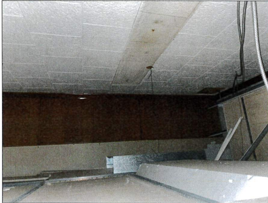
3 - View of sampled splined ceiling tiles
