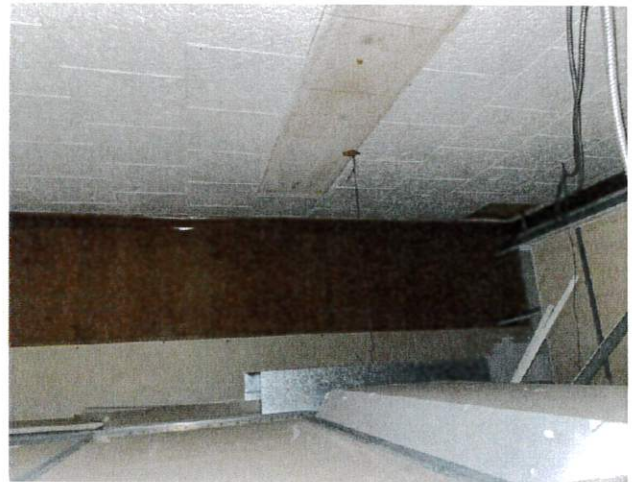
Sampled splined ceiling tiles
