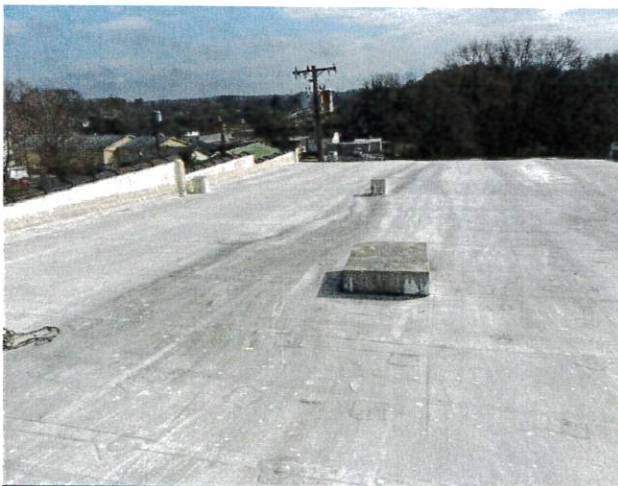
View of Lower Roof
