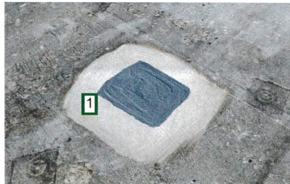
Repaired: Upper Roof Core (Location 1) permanent repair. Self-adhering membrane was placed over existing patch and sealed.
