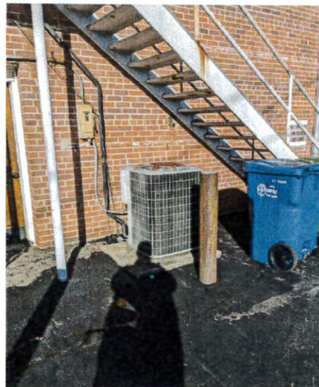
Air Handler #3/ Condensing Unit #3
