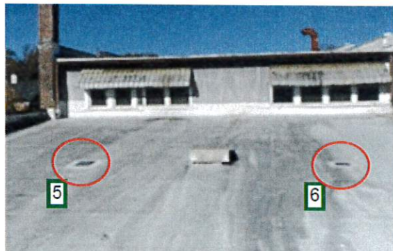
Repaired: Lower Roof Core and Lower Roof Puncture repair complete (Location 5 & 6). Self-adhering membrane was placed over existing patch and sealed.
