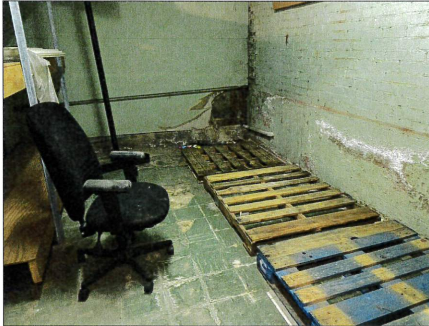
7 - View of basement storage room
