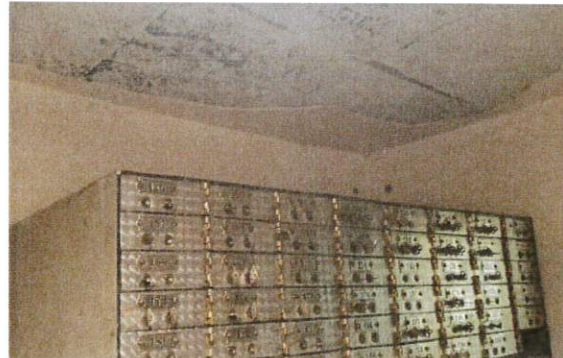
Concrete wall at the vault
