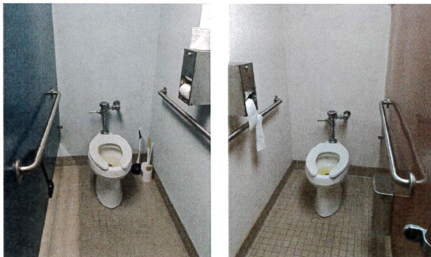
Main Level Men's and Women's Toilet
