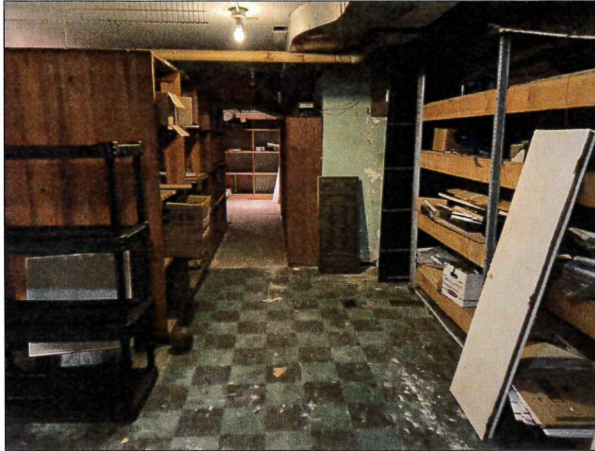
9 - View of basement
