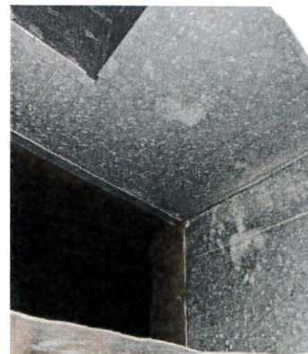
Exposed ductwork in basement with hole and no insulation
