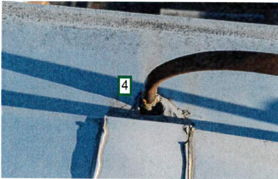
Existing: Upper Roof Conduit Penetration (Location 4).
