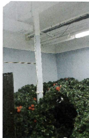
Basement at addition side
