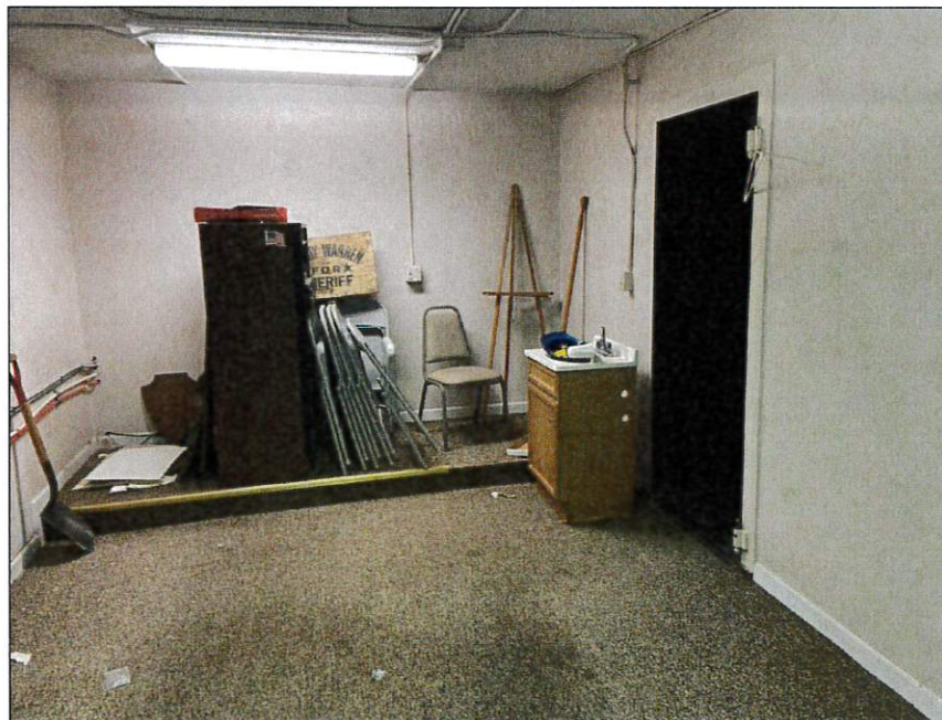
8 - View of basement safe
