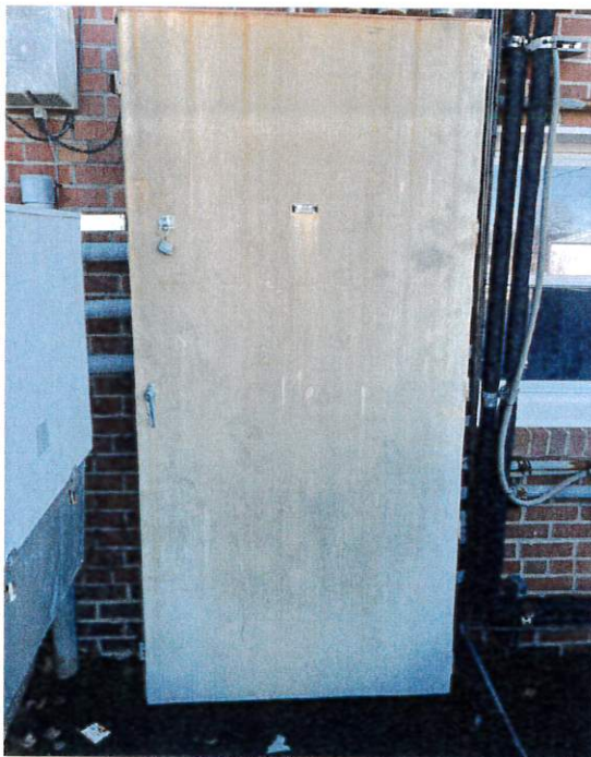
Main Distribution Panel
