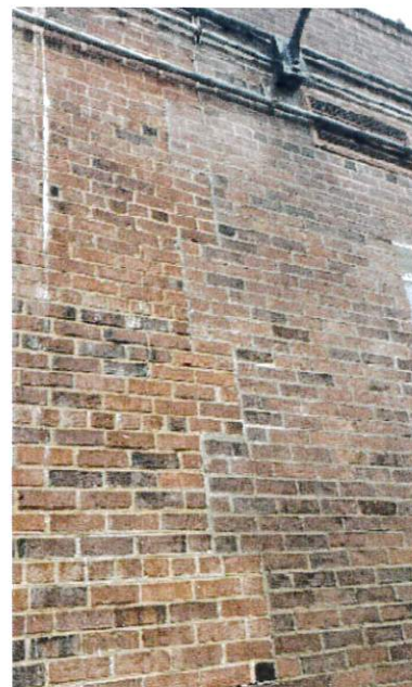
Joint at addition
