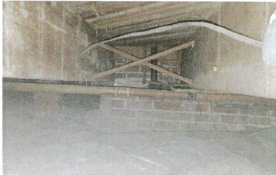
Floor Framing in basement bathroom
