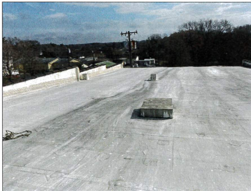
4 - View of lower roof
